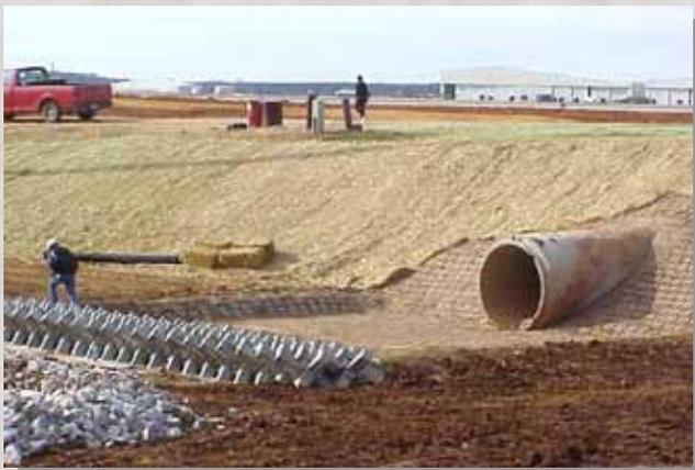
**PRODUCT:** Armortec ArmorFlex Class 50s Articulating Concrete Block (ACB) Units, Cabled mattresses and A-Jacks AJ-48 Concrete Armor Units
